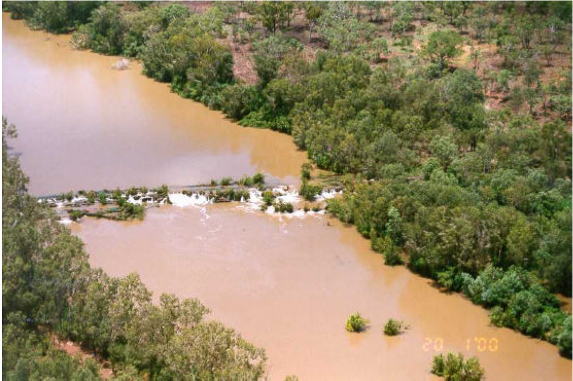
Photo A7 Aerial photograph of a tufa dam on the Flora River
